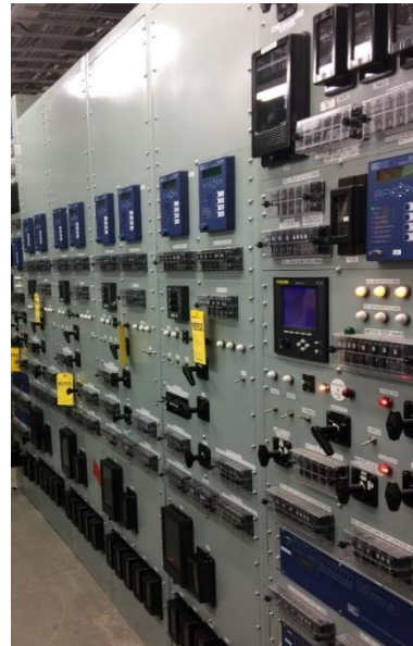
Modern Relay Panel (Single panel for relay and control functions)
