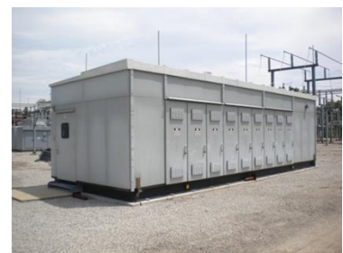
Two-Tier Switchgear
