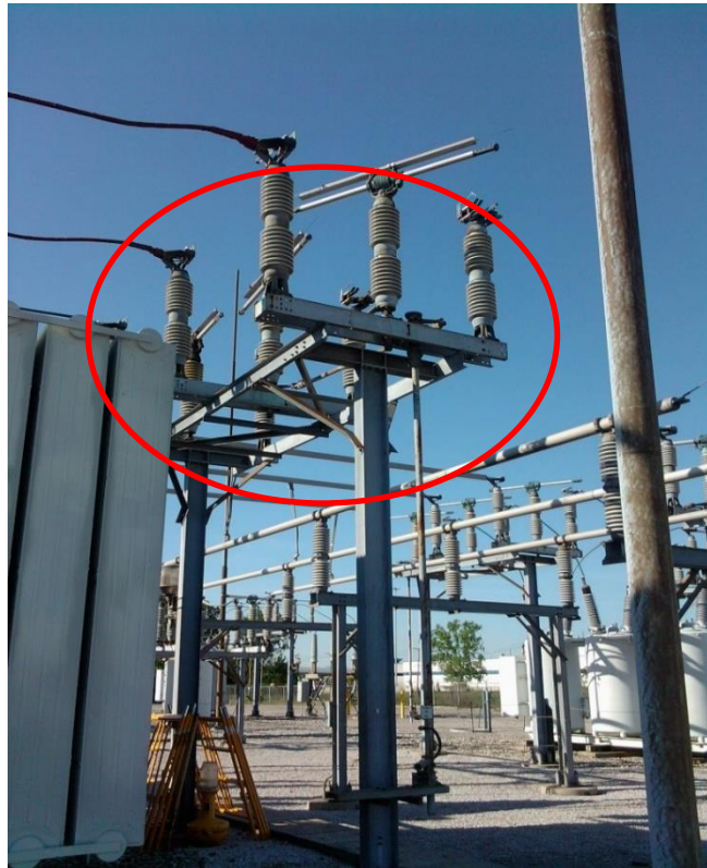
Exhibit 8.4.2 PM-40 Disconnect Switch
