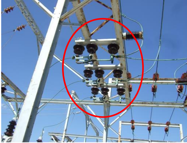
Exhibit 8.4.2 PM-40 Disconnect Switch
