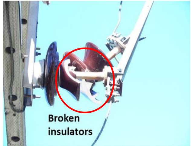
Exhibit 8.4.2 PM-40 Disconnect Switch
