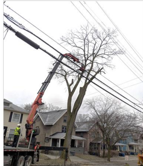
Removing a dead tree which has grown into the wires. Dead trees cannot be climbed, therefore specialty equipment is required
