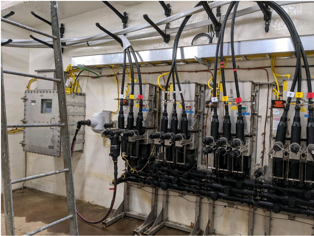
Exhibit 8.19.3 After Picture of a Service Vault
