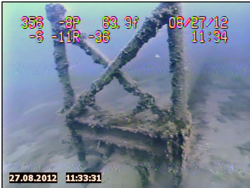
Figure 4 Frame Clipped from Enbridge 2012 East Leg Inspection Video
