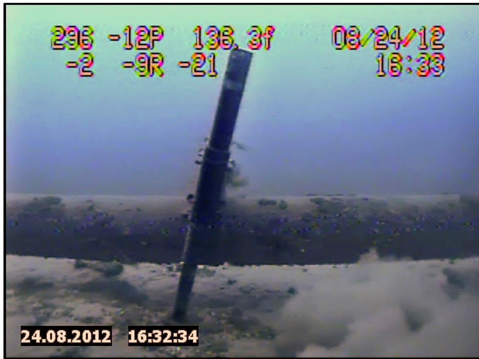
Figure 2 Frame Clipped from 2012 Enbridge West Leg Inspection Video
