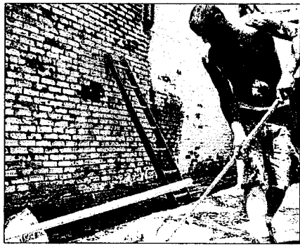
Matthew Dae Smith for the Lansing State Journal Daniel Boss of Lansing mixes concrete in Tuesday afternoon's heat. "We drink plenty of Gatorade and have an air-conditioned area we can take breaks in," he said.
