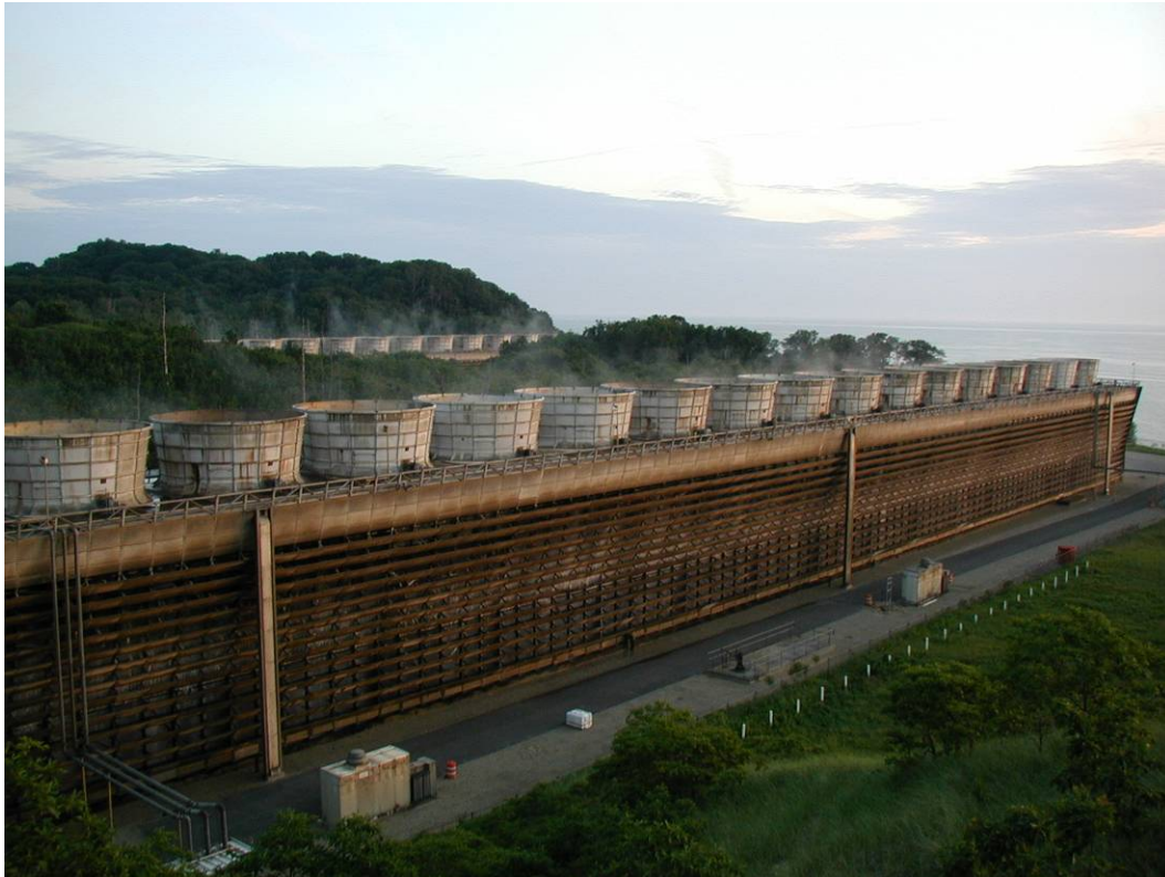
Figure 2-2: Palisades Cooling Towers
