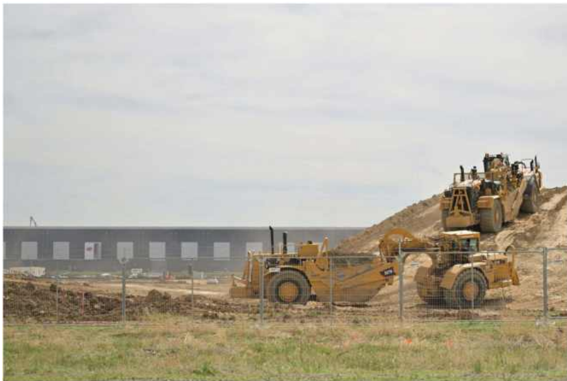
The construction site of a 65-acre data center on May 13 in Aurora, Colo. The new facility could consume as much electricity as 176,000 homes. Credit: RJ Sangosti/MediaNews Group/The Denver Post via Getty Images
