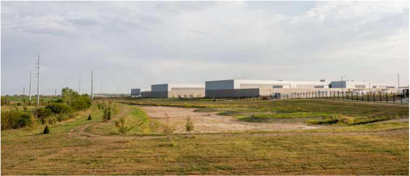
A view of the Sarpy County Data Center in Omaha, Neb. Credit: Misty Prochaska/The Washington Post via Getty Images
