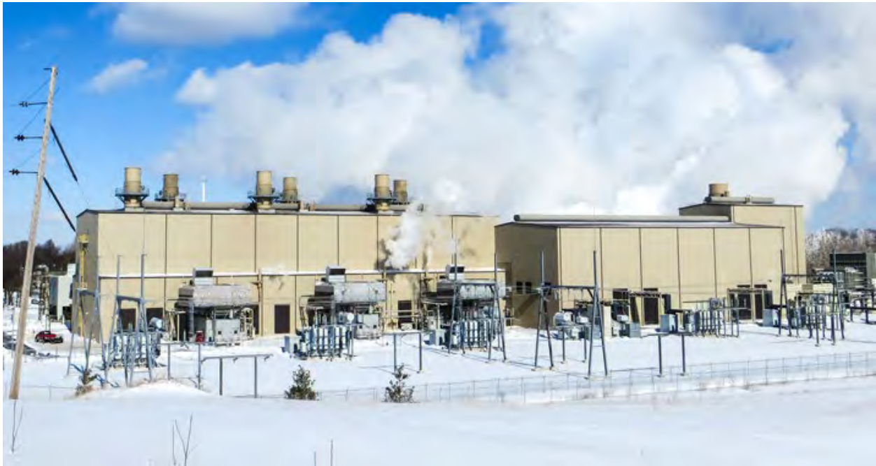
Figure 1. Jackson Generating Station.
