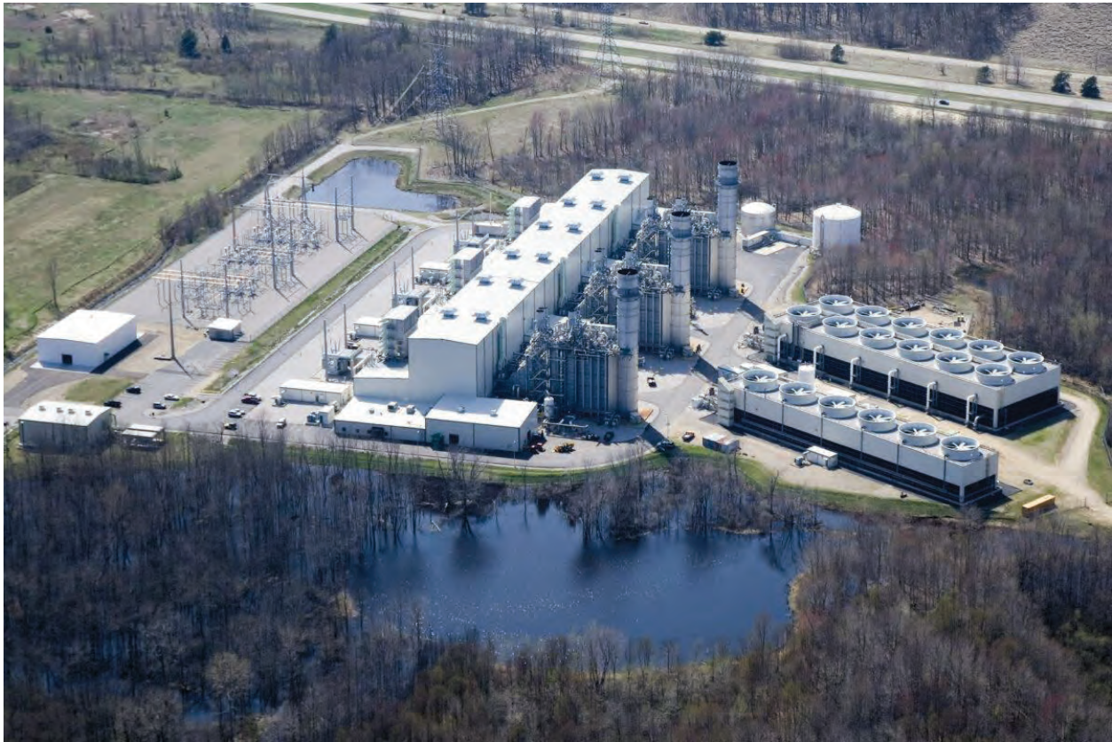
Figure 1. Covert Generating Station aerial view.
