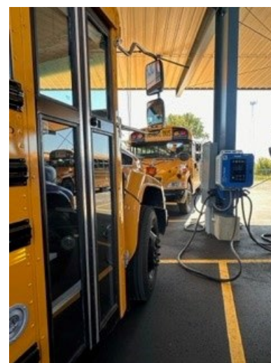
A school district installs 30kW Long-Duration DC chargers to power new electric school buses
