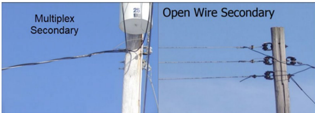
FIGURE 26 MULTIPLEX VS. OPEN WIRE SECONDARY
