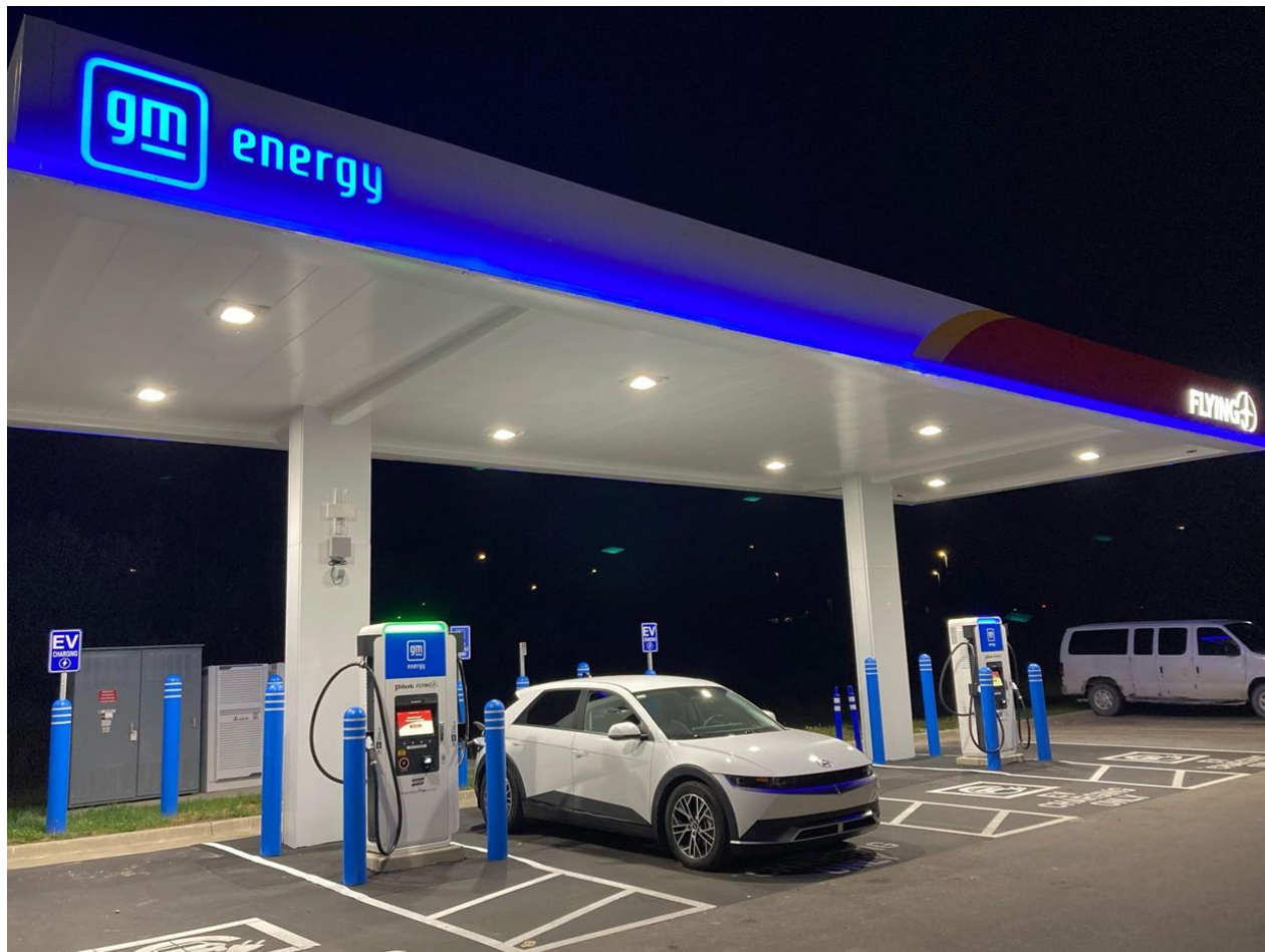
A fast-charging site in Saginaw supported by PowerMIDrive offers excellent lighting and a canopy
