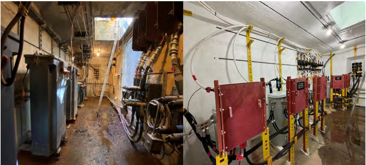
FIGURE 45 VAULT BEFORE AND AFTER RELIABILITY PROJECT
