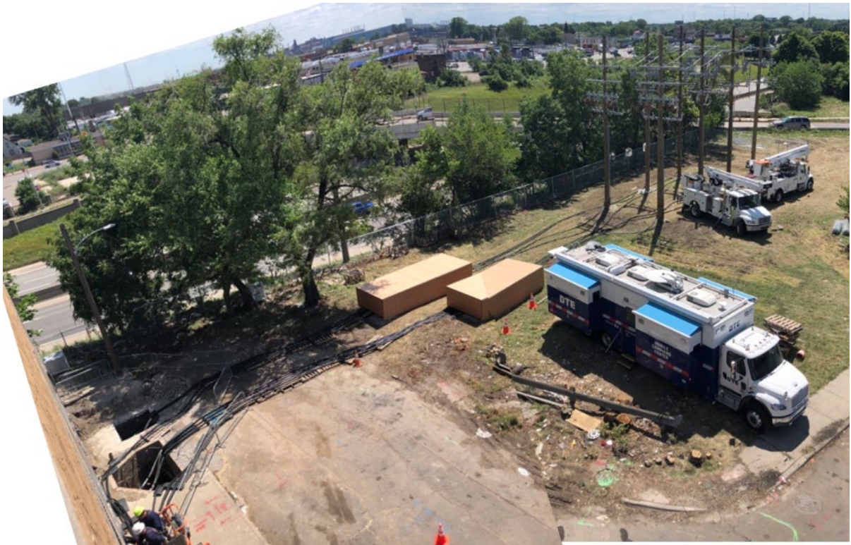
Figure 15. McGraw Substation – Temporary Pole Farm
