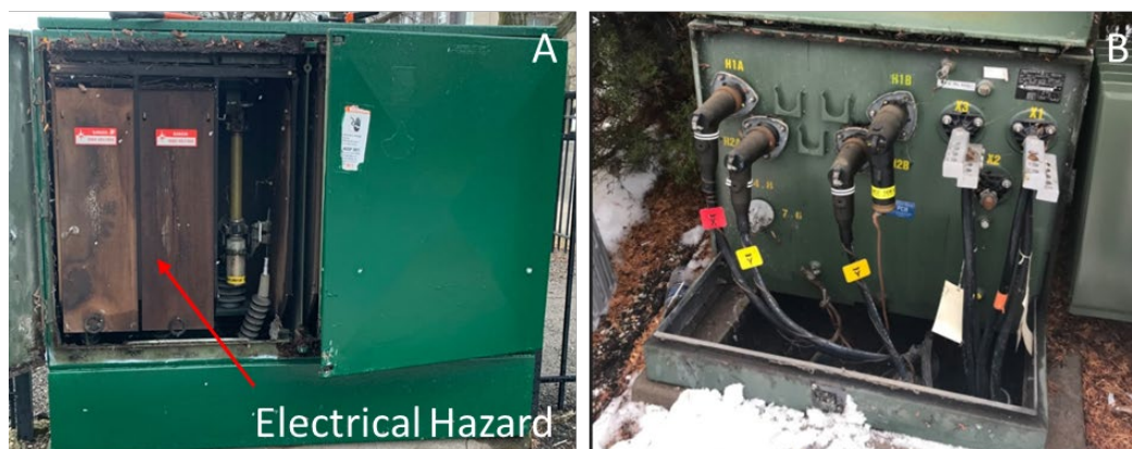
Figure 12. (A) Live-front and (B) Dead-front UG Transformer
