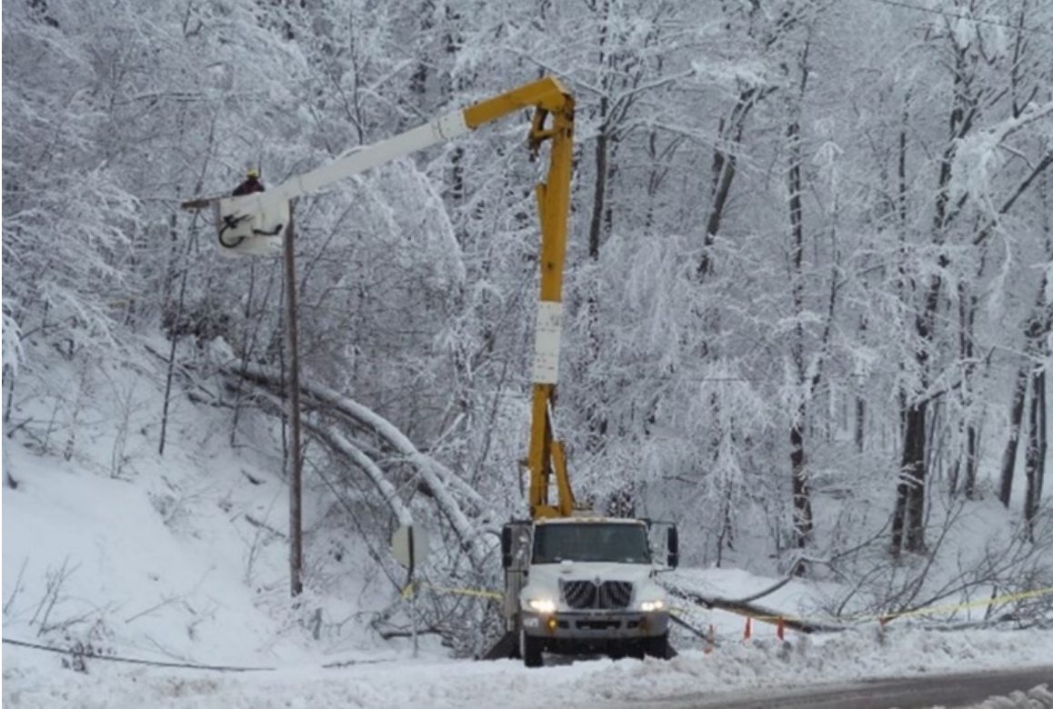
Effect of wet, heavy snow on trees and electric lines
