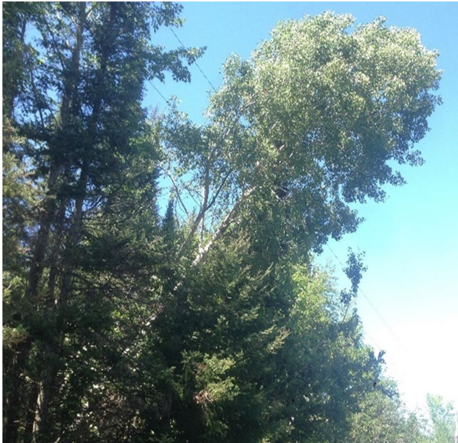
Healthy off-right-of-way tree towering over/falling into electric line
