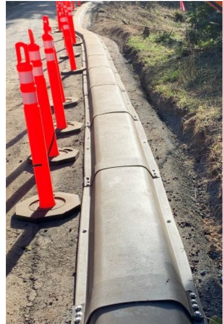
Example of a Ground Level Distribution System *Photo courtesy of Pacific Gas & Electric
