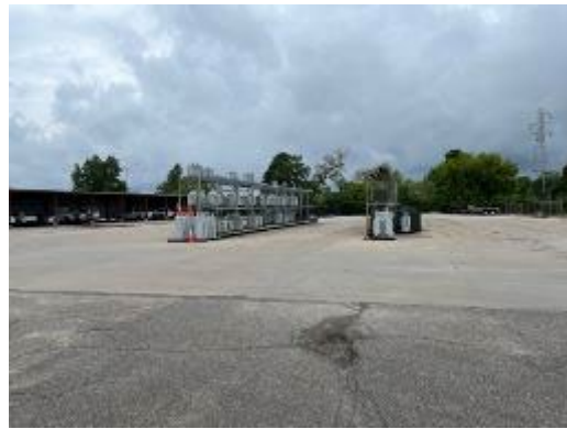
Cadillac service and isolator transformers
