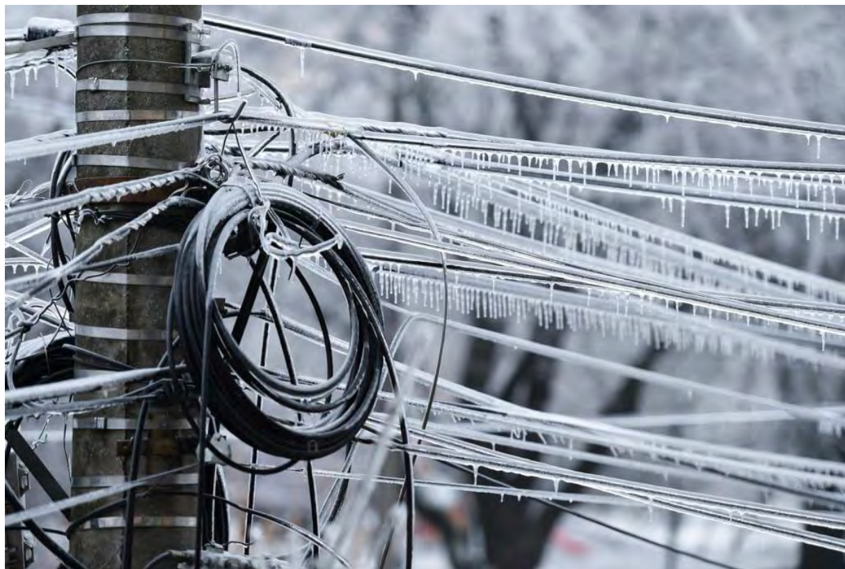
Ice on power lines is one reason for power outages. Credit: roibu
