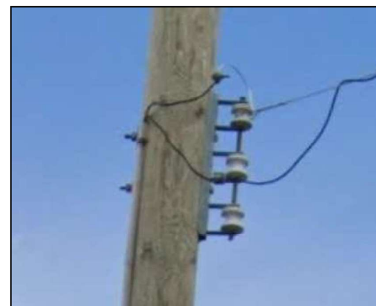
Acceptable Spool Rack
