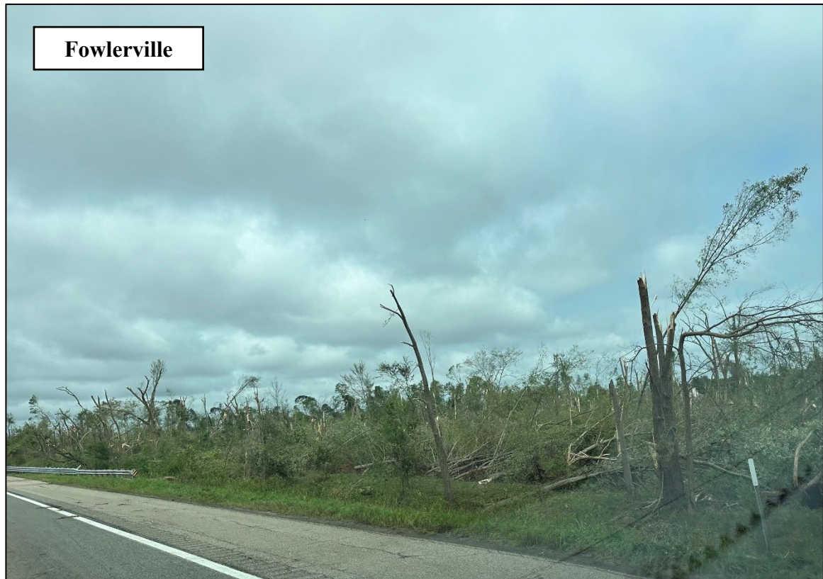
Figure 4 August 23, 2023 Storm Damage
