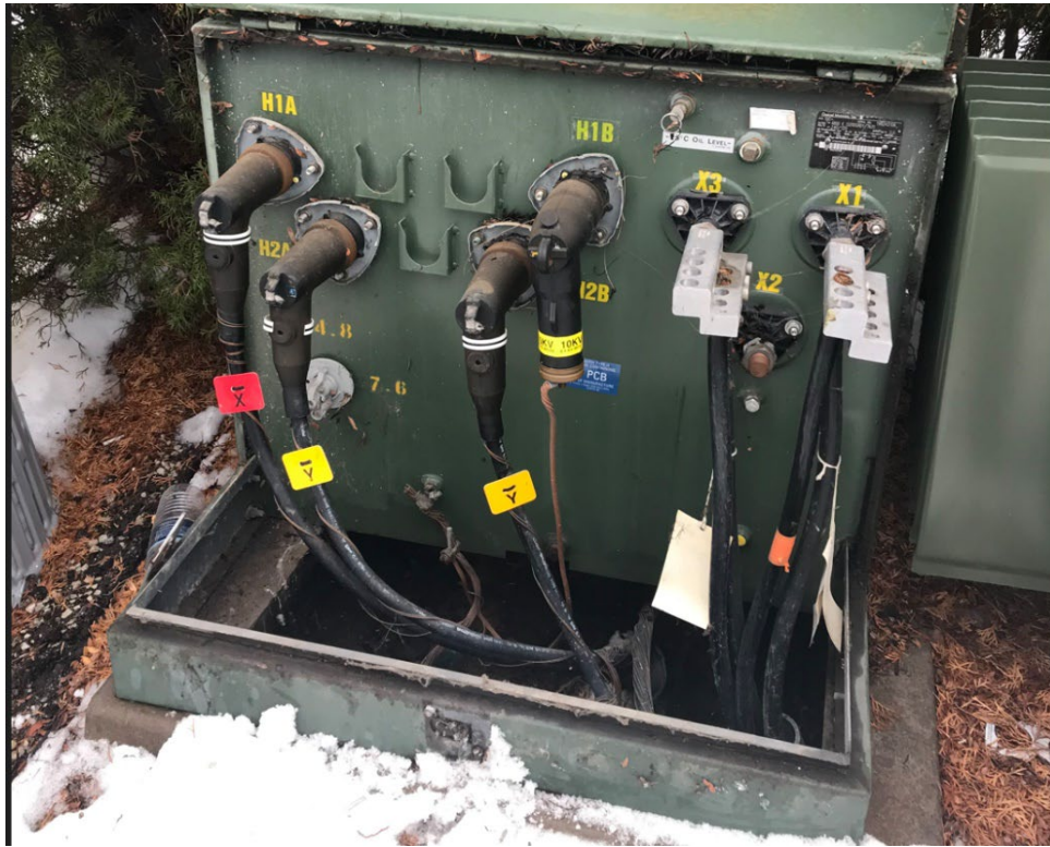
Figure 28. Dead-front UG Transformer
