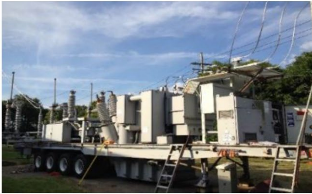
Figure 29. Portable Substation (left) & Mobile Generator (right)
