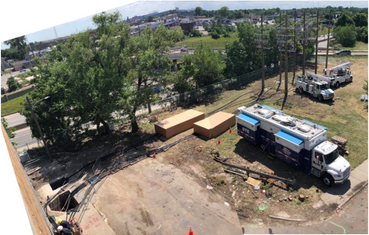
4 5 Figure 19. McGraw Substation – Temporary Pole Farm
