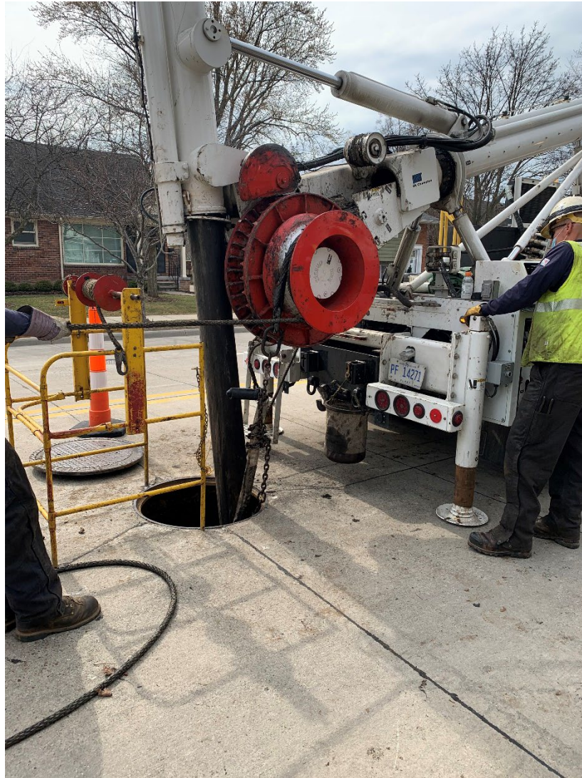
Figure 25. System Cable Pulling (Removal)
