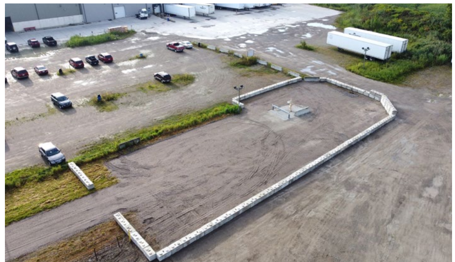
Well Site Protective Barriers - Figure 53
