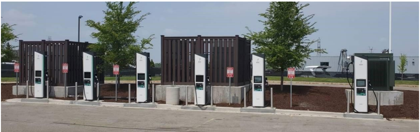
A string of six 350 kW fast chargers in Hudsonville
