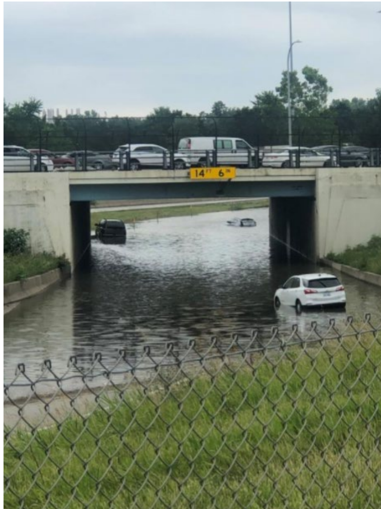
Figure 16. Flooding Near McGraw Substation
