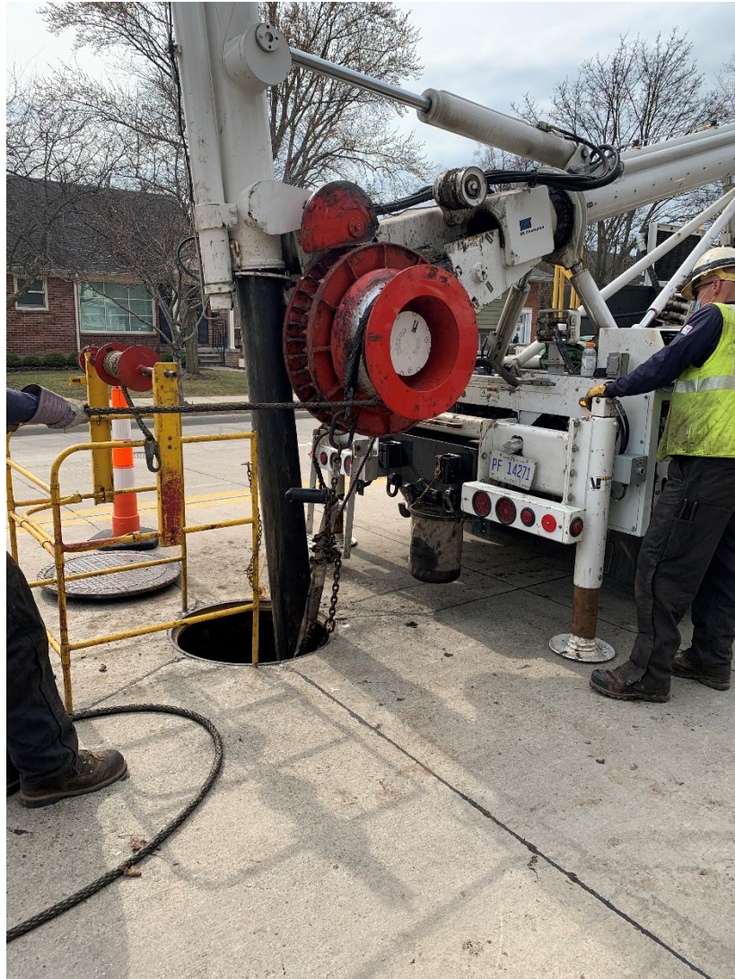
Figure 25. System Cable Pulling (Removal)
