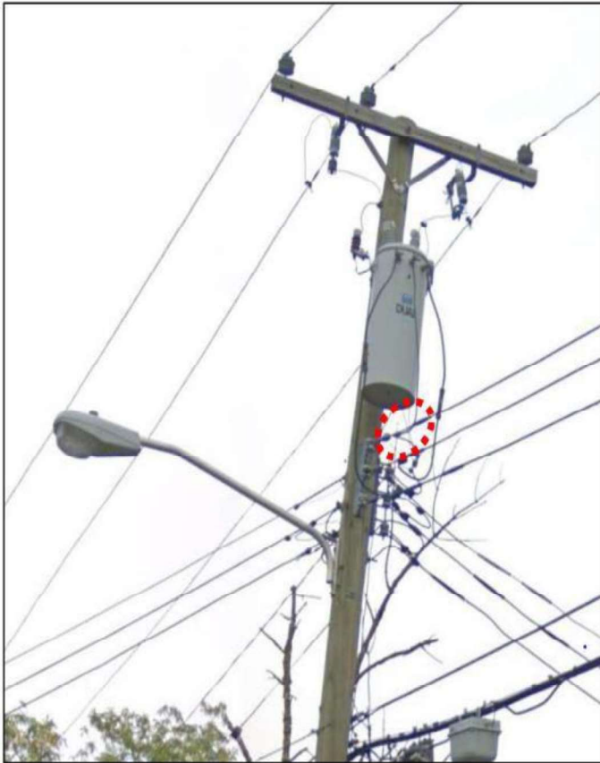
Acceptable Neutral Tap on Secondary
