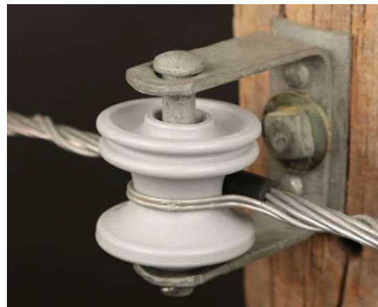
Acceptable Neutral Spool Assembly
