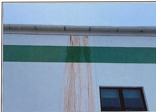
Water Roof Discoloration Primary Building
