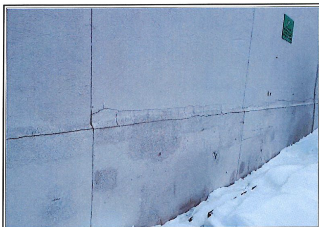
Cracking Concrete Finishing Primary Building
