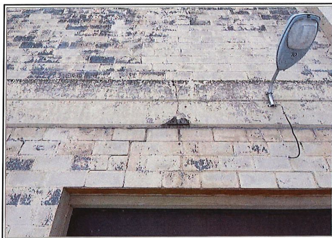
Peeling Paint/Cracking Concrete 3-Story Storage Building
