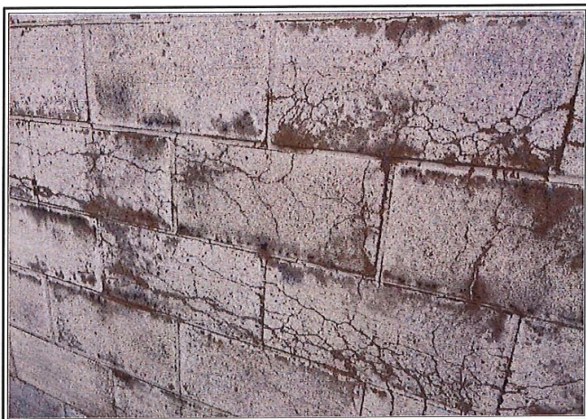
Cracking Block 5-Bay Garage
