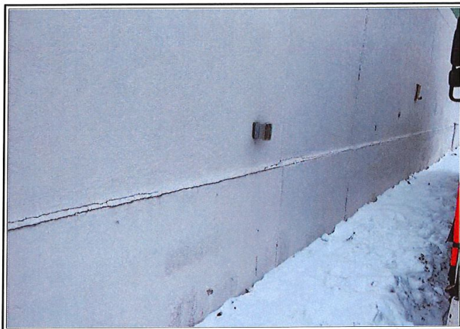
Cracking Concrete Finishing Primary Building
