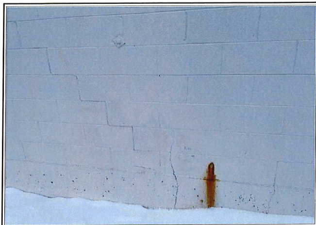
Joint Crack Primary Building
